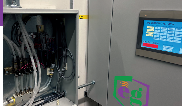
enVgrow's CO 2 flow station and controller with Gas settings in every zone.
